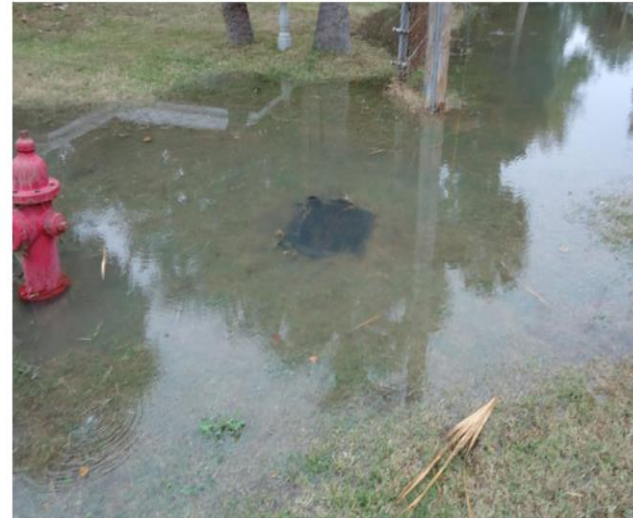
FIGURE 4.6: STORMWATER DRAIN WITH SALTWATER DISCHARGE DURING KING TIDE, NOVEMBER 14, 2012
